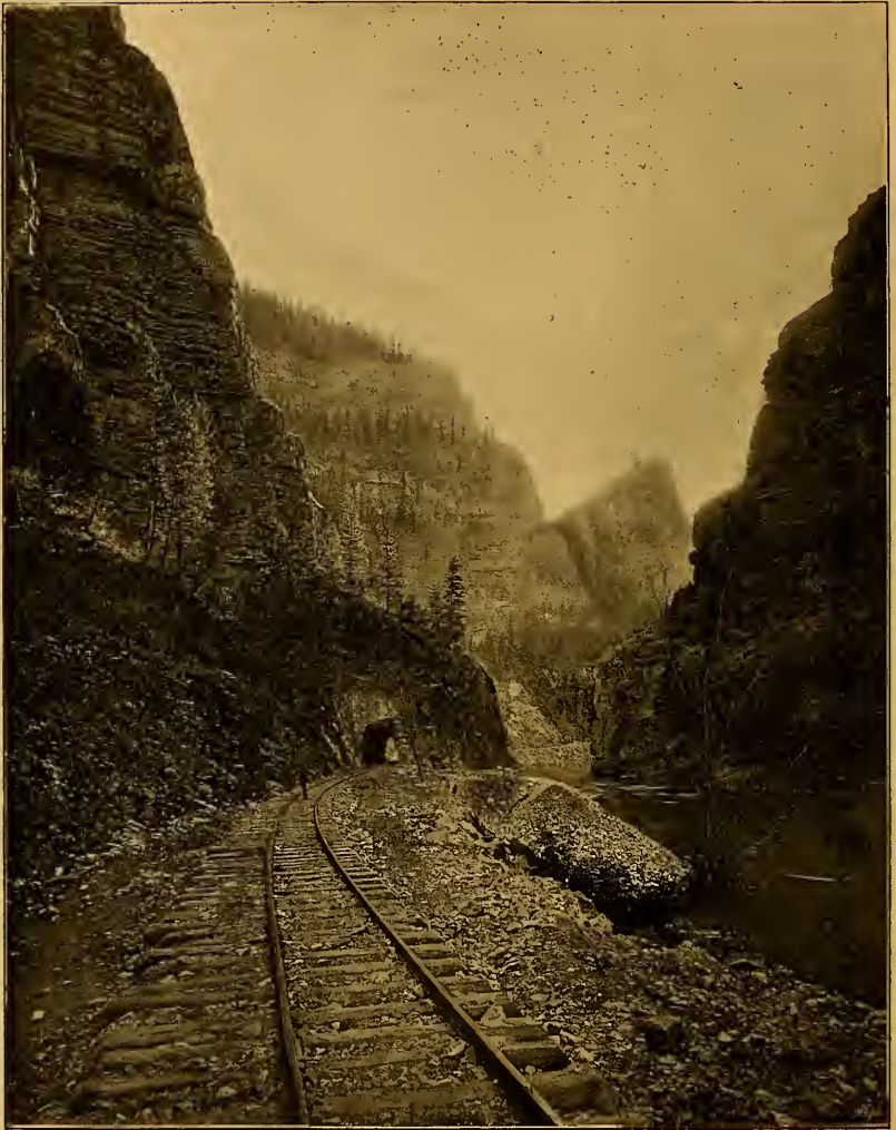
FIG. 46. TUNNEL ON THE GRAND RIVER CANON.
